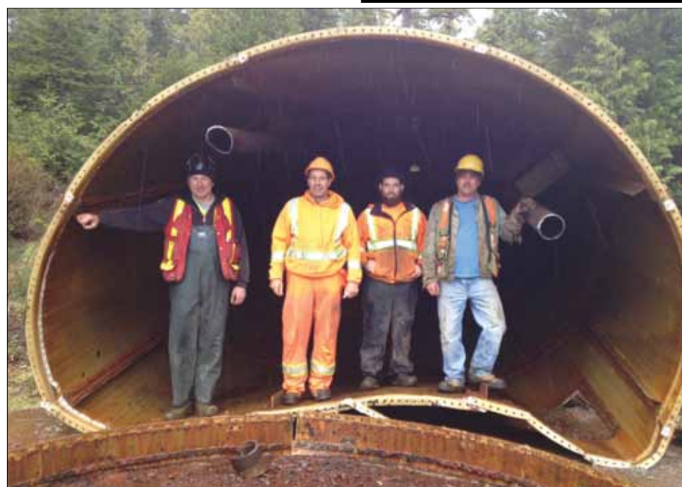
Above: the construction crew doing the road work for the sewer and water upgrades were also contracted to take down the old water tower. Mission accomplished, here they are pictured in the bottom of the tank.
