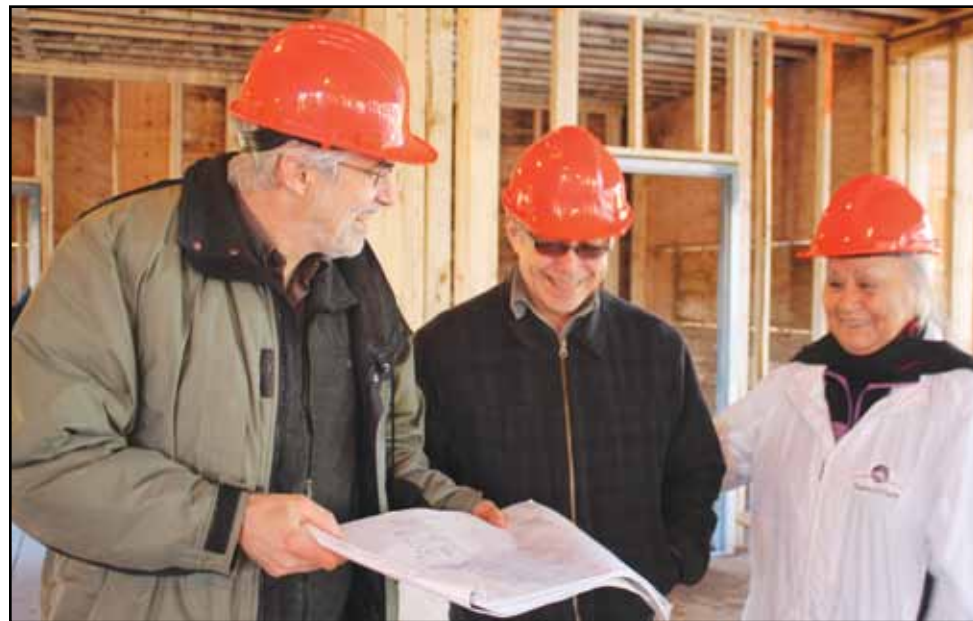
Yuułu?il?ath Legislature members Geraldine Touchie and Alan McCarthy take a look at plans with architect Scott Kemp during a site visit of the new community centre.
